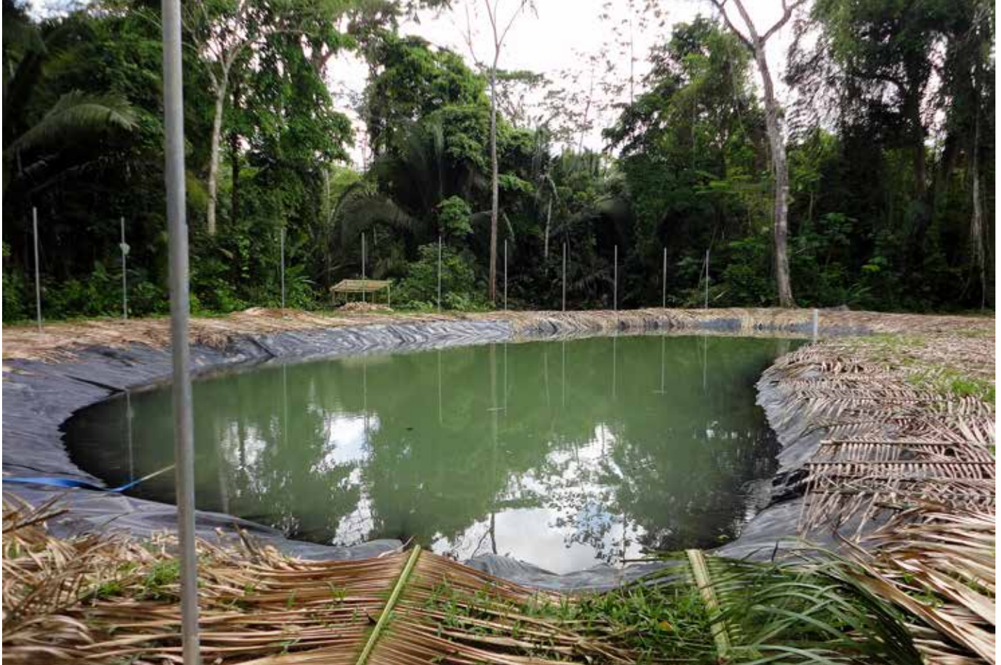
One of the two breeding ponds is now holding water, thanks to the artificial liners. Note the 4-inch PVC vertical pond drain which can be swung manually to adjust pond levels to the desired depth. Cohune thatch palm leaves have been placed around the perimeter of the ponds to mitigate any erosion that might take place during the coming rainy season and until natural vegetation takes hold. PHOTO CREDIT: WILLIAM GARCIA
