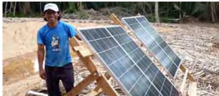
Tom Pop, who supervised the breeding facility construction, stands with the solar panels that will power the well pump. PHOTO CREDIT: JACOB MARLIN
